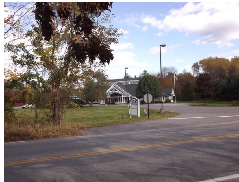
Plaistow Town Library—Note Absence of Pedestrian Access fro Main Street
