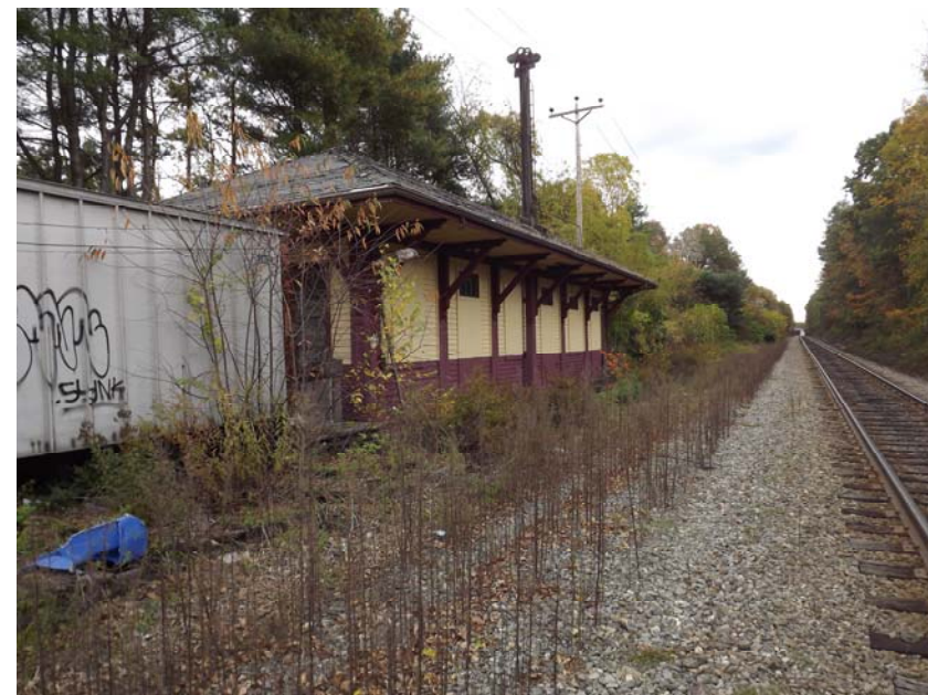
Privately Owned Railroad Station Building—Potential trail head/visitors building or farmers market.
